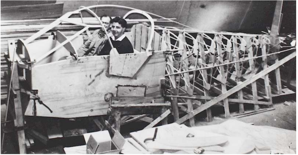
Tom Webb and Trevor Sloane sitting in the partially completed fuselage.
